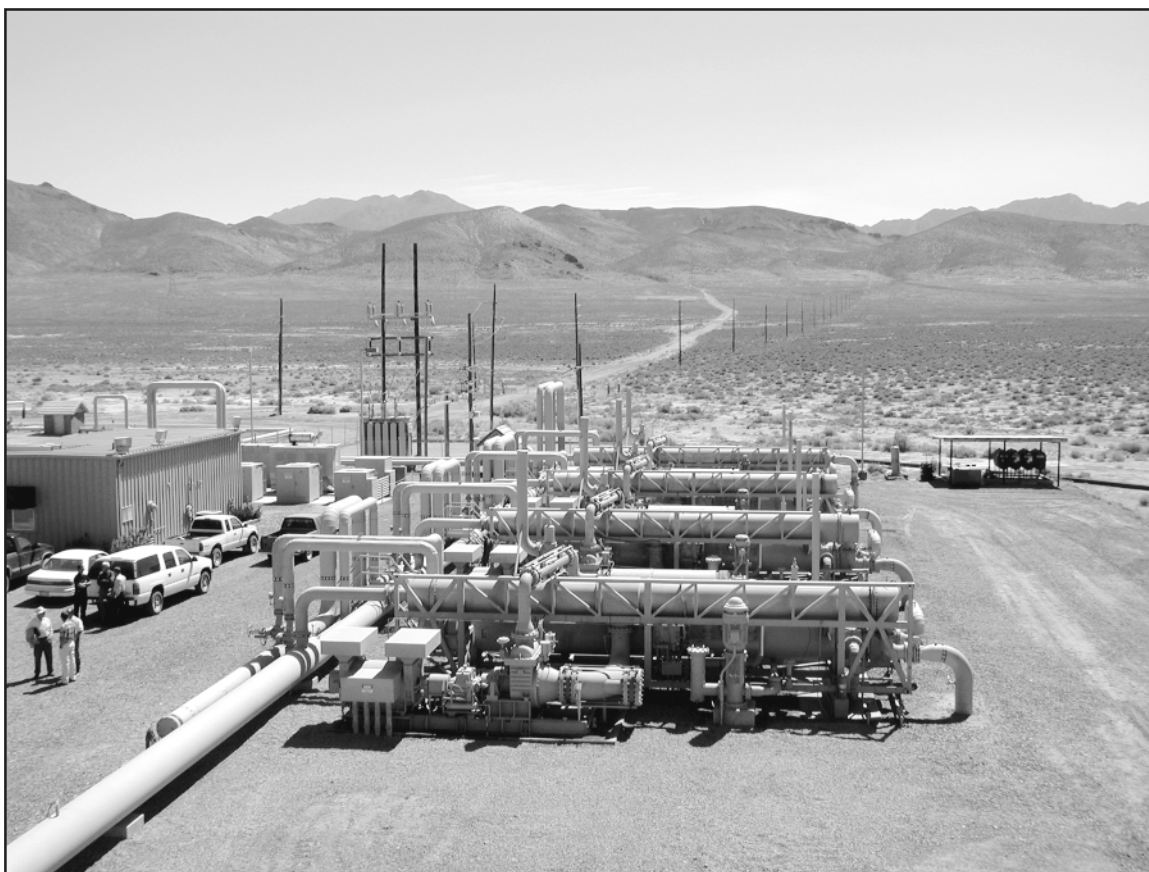
Binary generation units at the Empire Farms geothermal plant and garlic and onion drying facility. Photo by Larry Garside, 2001.
