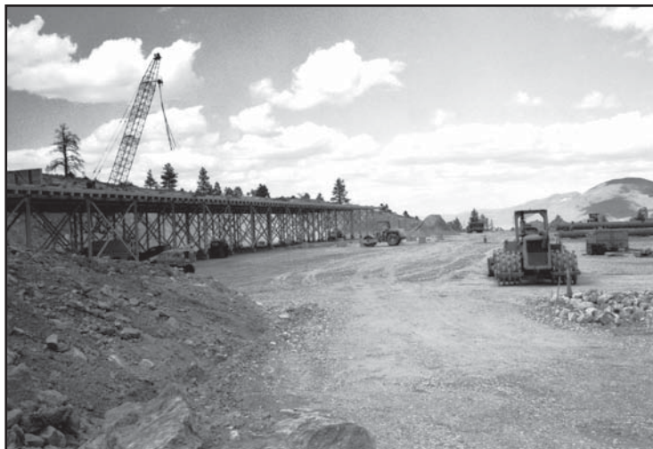
Construction of the Galena project at Steamboat Hot Springs is underway. This photo shows the ongoing construction of one of the two banks of condenser towers that will be part of the new geothermal power plant. Photo by R. Hess, June 2005.
