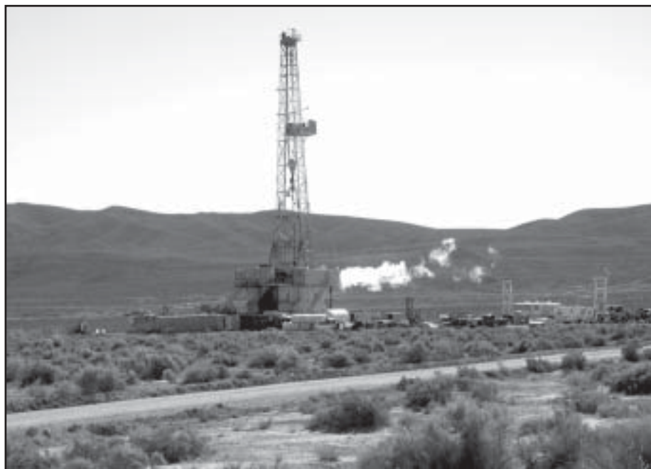
C. and L. drill rig at Brady Hot Springs drilling geothermal observation well 88-11 during the summer of 2004. Photo by Larry Garside.
